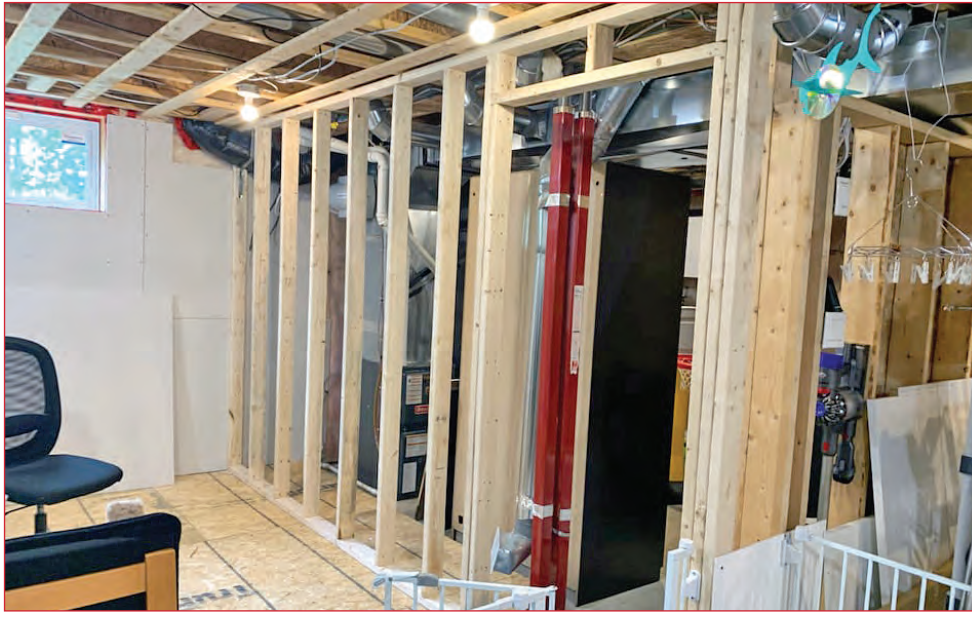
Some indoor work completed by Local 613 Property Maintenance. Courtesy Photo
