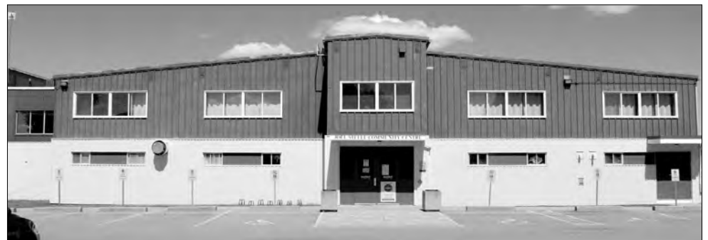
The Joel Steele Arena in Winchester will be getting a new chiller, a crucial part of their ice making process.
