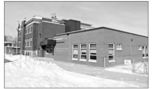
The Winchester Public School day care construction project is expected to start in the spring. Morin Photo
